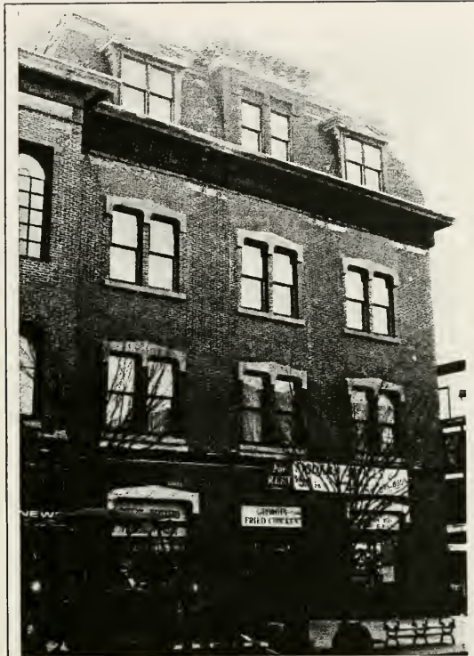
Figure 7. Old City Hall, 2-8 North Broad Street Trenton, NJ. North elevation. The outline of the previous glass block is apparent around the windows on the second and third floors. Photograph by Scott Doyle.
